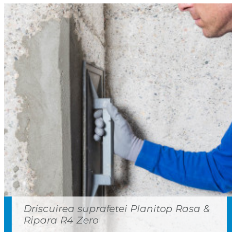
Aplicarea Planitop Rasa & Ripara R4 Zero
